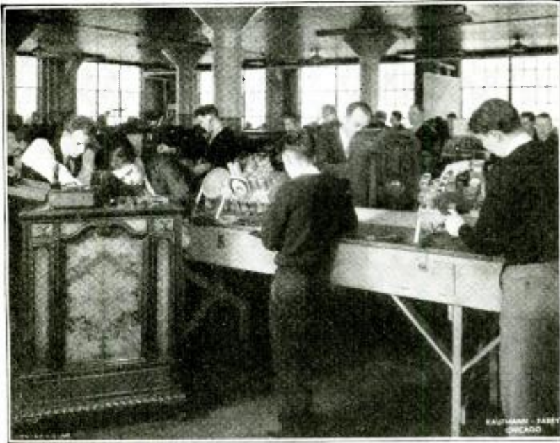
STUDENTS BUSY AT WORK IN GREAT COYNE SHOPS
